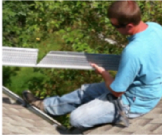
To fabricate a corner, a notch is cut from the guard up to the back wall.
