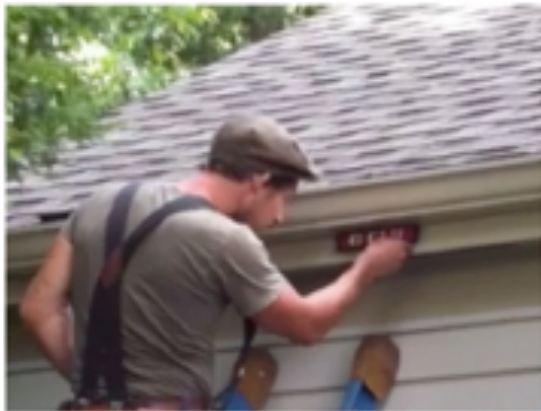
Gutter drainage angle is checked prior to anchoring the gutter.
