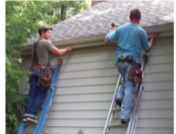
Working together, the installers anchor one end of the gutter assembly.
