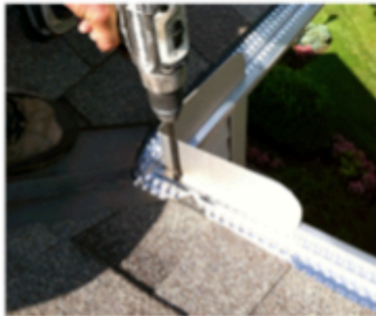
Zip screws secure the front edge of the guard to the gutter.
