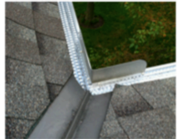
Notice the corner splash deflector is secured on top of the Perma Flow guard to assure good drainage.
