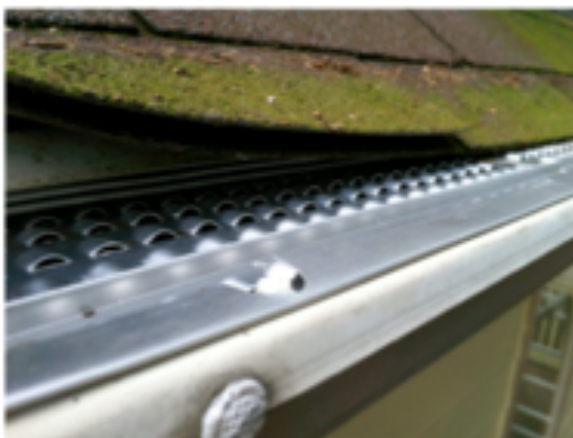
For tight spaces, the back wall may be folded down to create a flatter profile.
