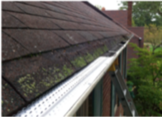
Perma Flow guard section installed on top of a spike and ferrule gutter.
