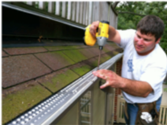
Securing the guard using 1/2" zip screws.
