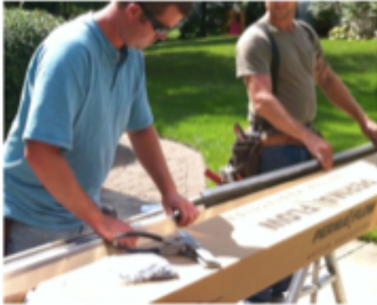
Sections of Perma Flow guard are angled and snapped into position on the gutter.
