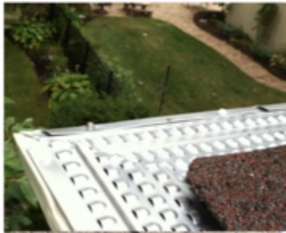
Another close-up view showing two pieces using a 45 degree miter cut overlap.
