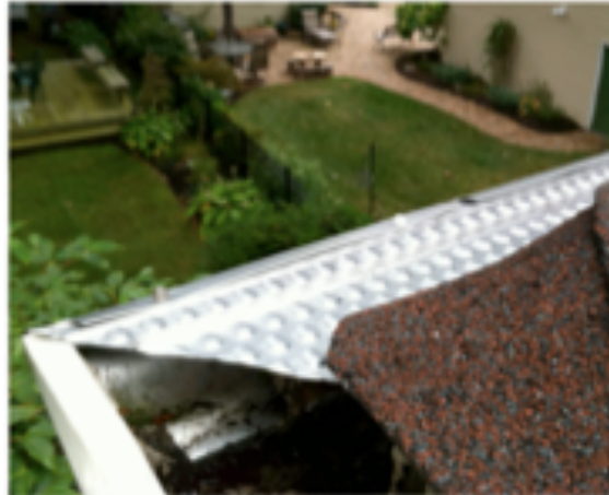
The first piece of guard is secured to the gutter front edge.
