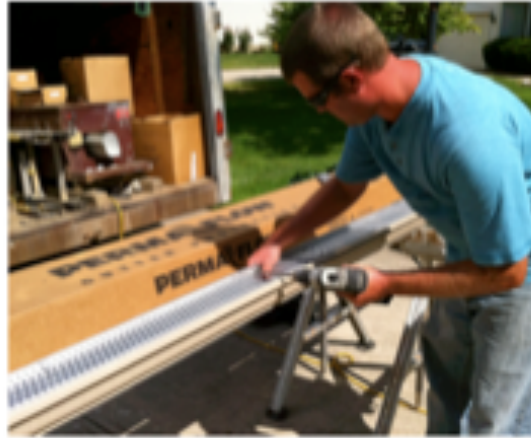
Screw anchors are put into position every 24" using the factory pilot holes.
