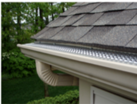
The gutter is hung correctly with the drip edge in front of the Perma Flow guard.
