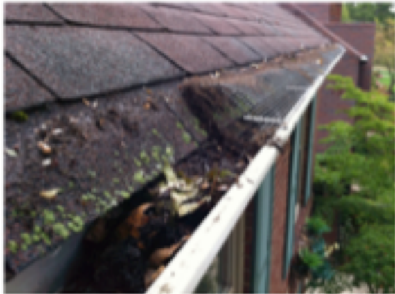
A before view of the existing wire guard and the amount of debris that has collected.
