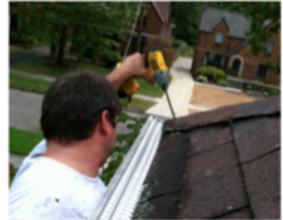
Screw fasteners secure the corner section in place.
