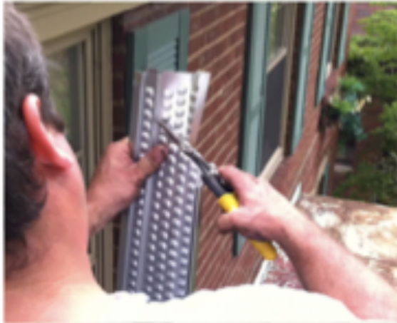
The installer is hand cutting a 45 degree miter angle.
