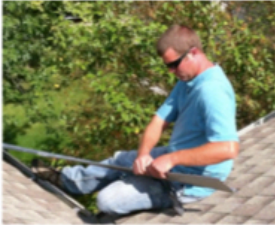
The installer is hand crimping a length of guard due to the tight working area.
