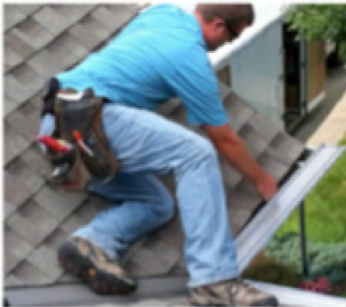
The corner assembly is tucked into position.
